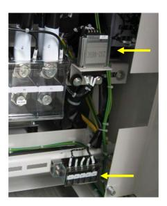
2. The COM-SAN interface option, together with earthing conductor (PE) – length 70 cm.
