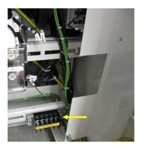
4. Place an additional DIN-rail (length 6 cm) as shown:
